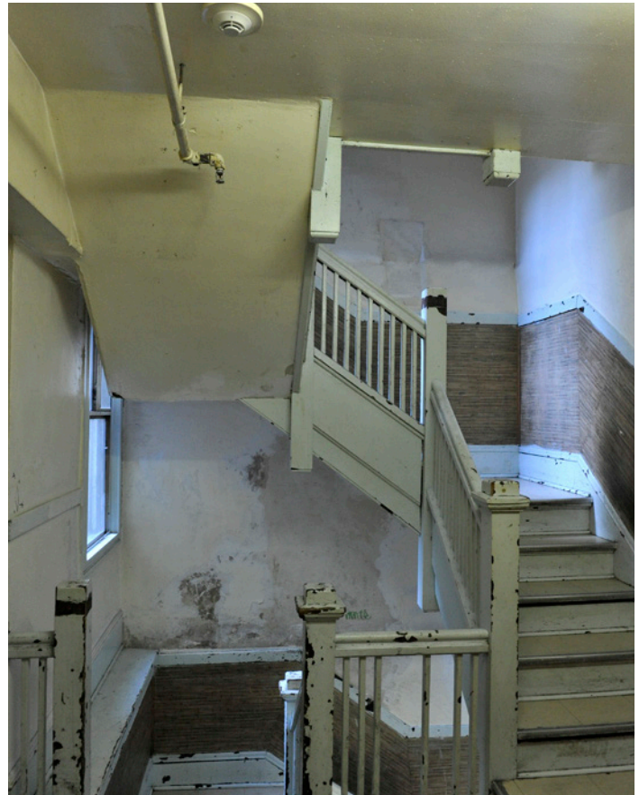
Gastown Hotel stairway before renovation
