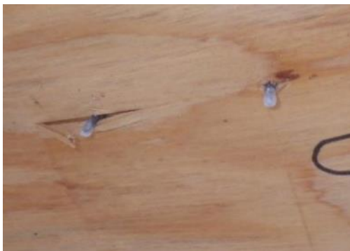
Figure 2.14 – Frost on nail heads of South facing roof slope on morning of January 2, 2013
