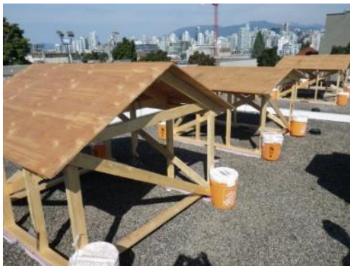
Figure 1.7 - Roof huts under construction with plywood sheathing installed
