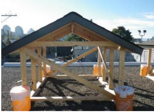
Figure 1.18 – Overview of 6:12 roof hut South (left) and North (right) slopes
