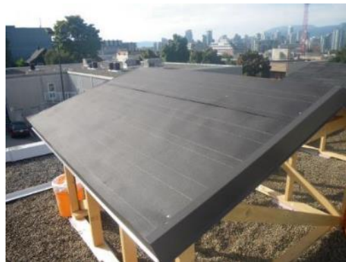
Figure 1.8 - #15 roofing felt underlay and perimeter flashings installed
