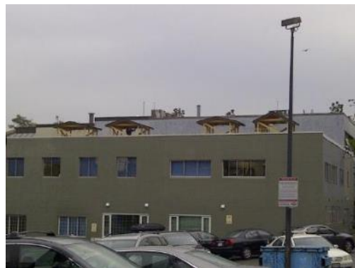
Figure 1.12 – Exposure of roof huts on top of 2 storey commercial building roof-top. From left to right: 3:12, 4:12, Control (3:12), and 6:12
