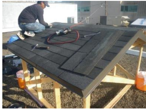
Figure 1.10 – Three-tab asphalt shingles being installed by roofing contractor
