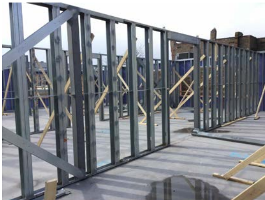
Figure 4-1: CFS system in platform-type construction (left) (summitdb.com, 2021) and schematic detail for platform-type construction (right) (Ccssbi, 2002)
