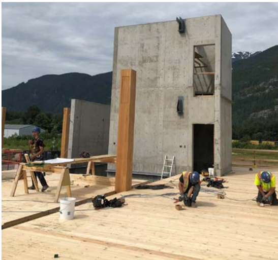
Figure 3-1: LLRS with concrete core – photo credit Hercend Mpidi Bita (left); and with steel braces – Photo credit Omer Mohammed (right)
