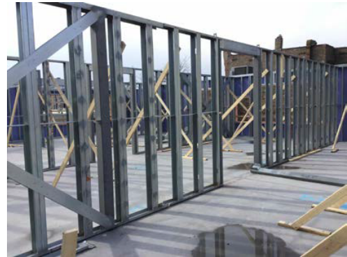
Figure 3. CFS system in platform-type construction (summitdb.com, 2021)
