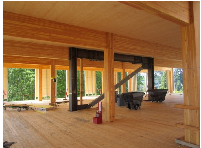
Figure 3-1: LLRS with concrete core – photo credit Hercend Mpidi Bita (left); and with steel braces – Photo credit Omer Mohammed (right)
