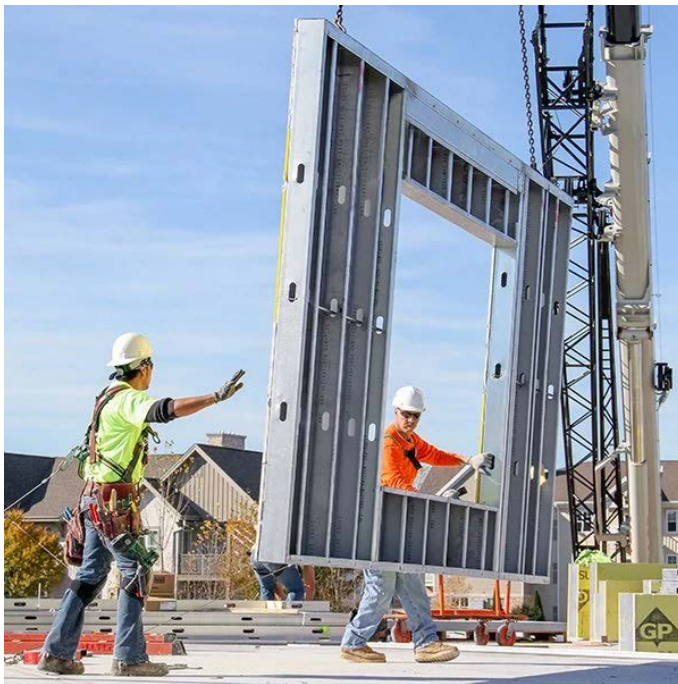
Figure 5-3: Panelisation of CLT/CFS structural components: CLT floor panel (top) – Photo Credit Kattera; and CFS wall (Walltechinc, 2021)
