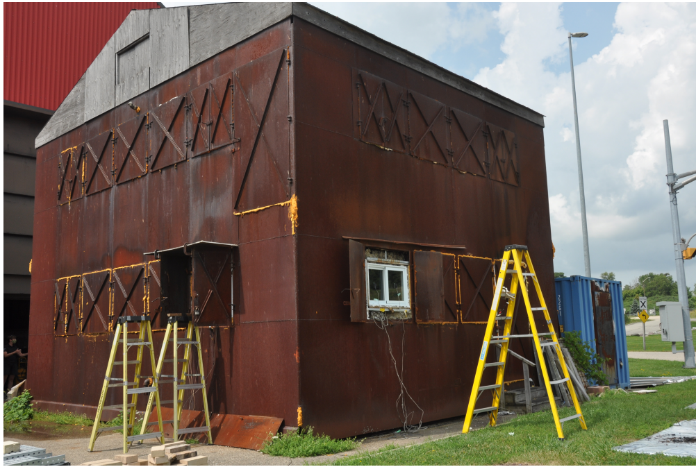
Figure 1: External view of the burn house structure.
