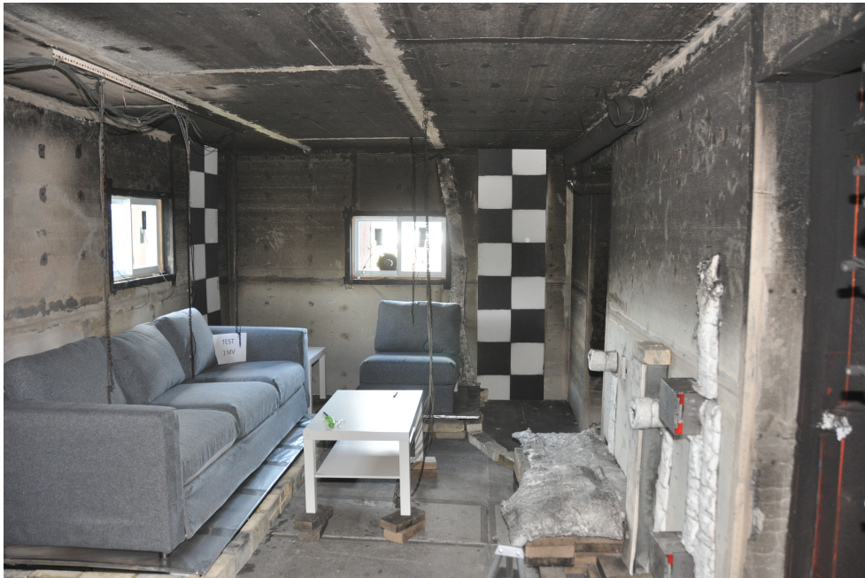
Figure 3: View of the fire room setup prior to a test.
