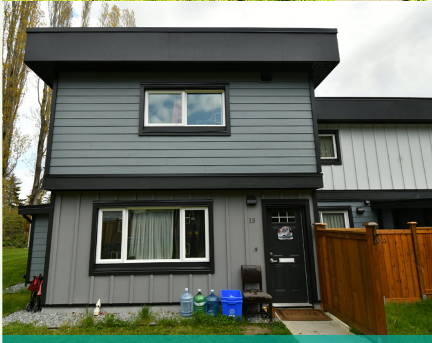
Edge Place Remediation Project – before and after
