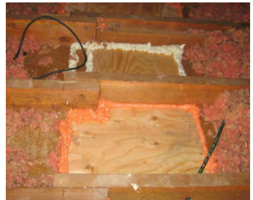
Spray foam around the edges of a cover, sealing it to surrounding joists and ceiling gypsum board.
