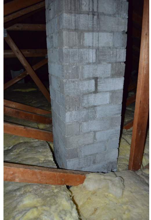
Masonry chimney in an attic.
