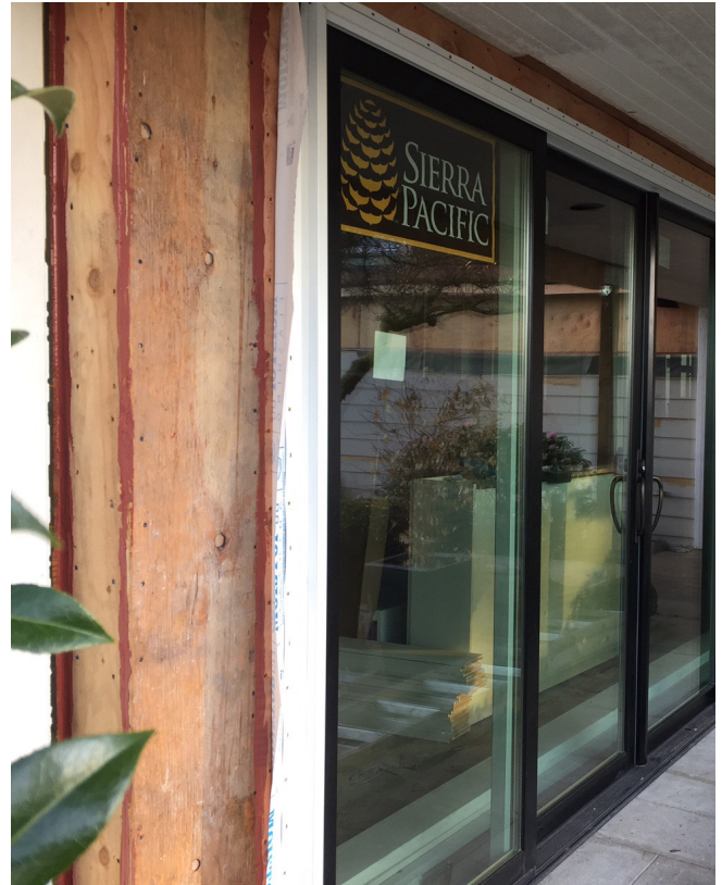
Replacement doors and windows are installed before the exterior insulation. For this project the air barrier approach was sealing all the gaps of the existing plywood sheathing.
