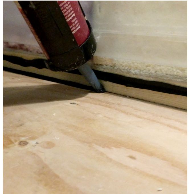
When polyethylene sheet is used as the interior air barrier, sealant is installed between the polyethylene and the bottom plate and between the bottom plate and the floor sheathing to ensure airtightness.
