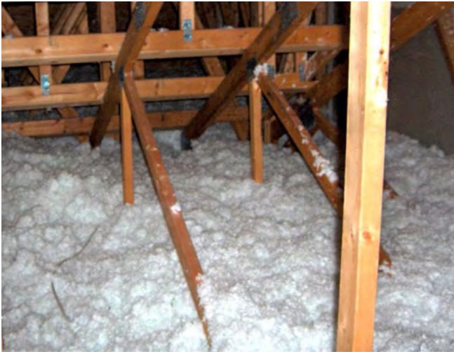
Blown-in attic insulation
