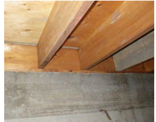
Exposed below-grade wall at floor rim joist.
