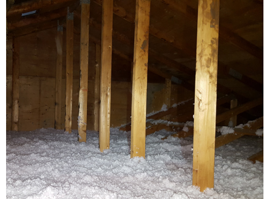
Gable end wall.
