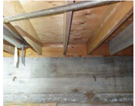
Uninsulated crawlspace interior walls and floor.
