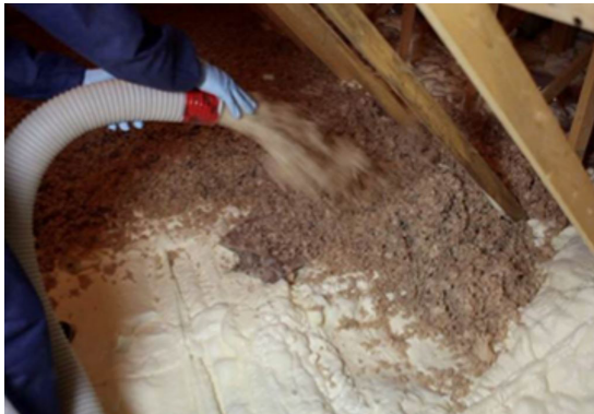
Insulation retrofit of an attic using blown-in cellulose added after air sealing and insulating with polyurethane foam.
