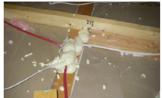
Top plate penetrations sealed with spray foam.
