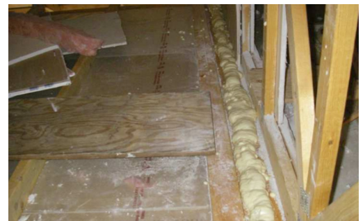
Spray foam installed over top plate joint.
