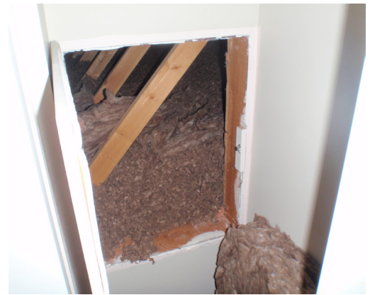
Access hatch at knee wall.
