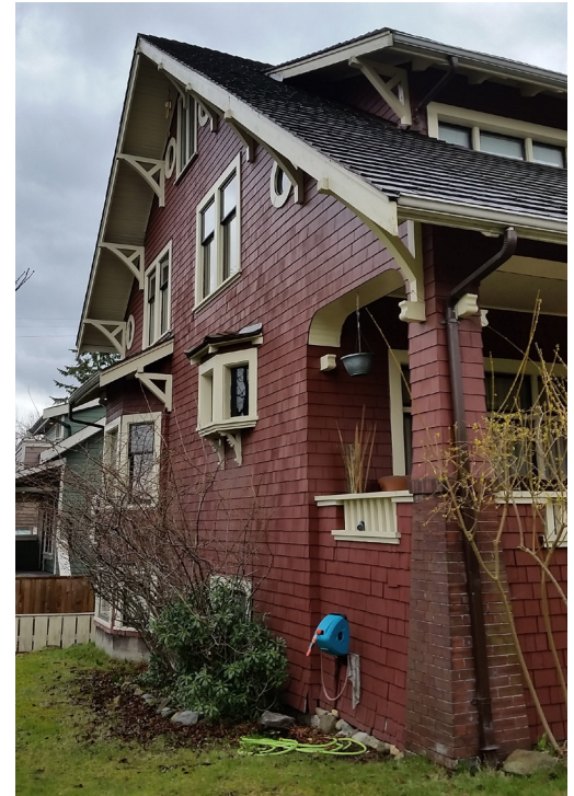
Older homes may have little or no existing insulation in the stud cavities.
