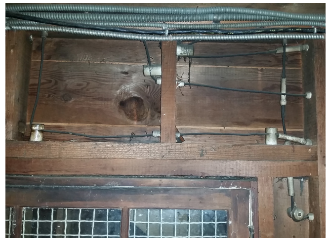
Knob-and-tube wiring.
