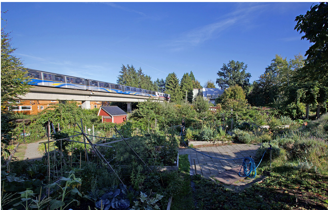
Figure 1. Future location of Vienna House
