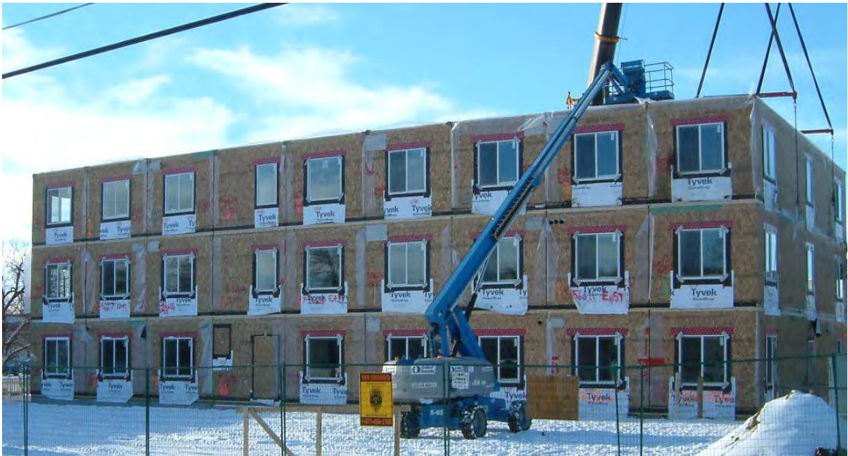
Figure 29: Canora Place: 27 Modules Set at -32 Degrees Celcius
