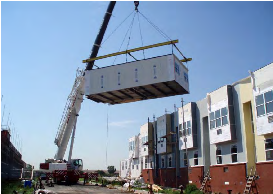
Figure 27: Nehemiah Spring Creek's over 800 homes, NYC's First Modular Social Housing
