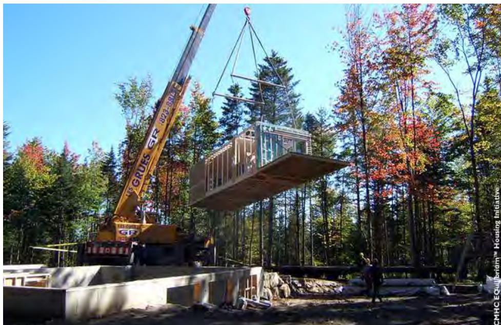
Figure 18: First ÉcoTerra™ Module Installed on Poured-In-Place Basement
