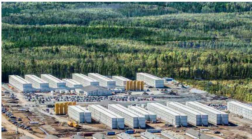
Figure 36: 15 Three-Story Buildings in 4 Months: Fort McMurray, Alberta
