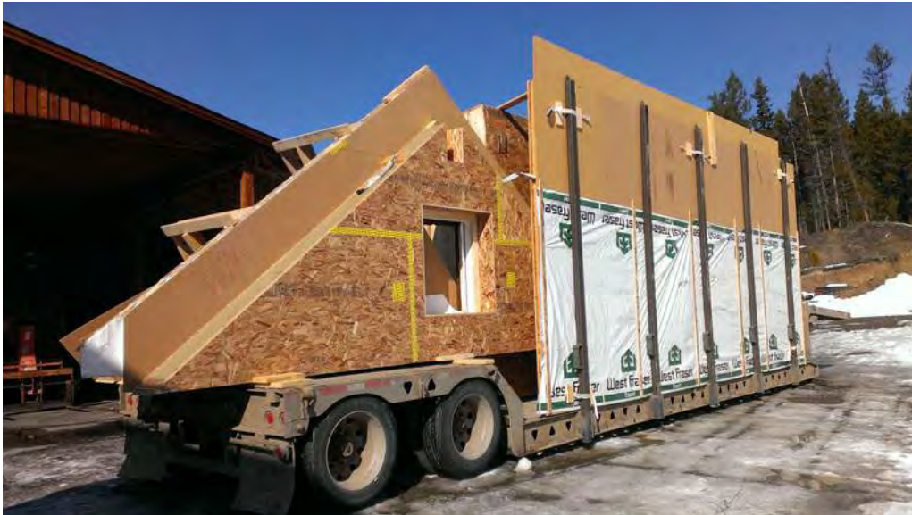
Figure 25: Truck Delivery of Fort St. Johns Passive House, Including Modular Roofing
