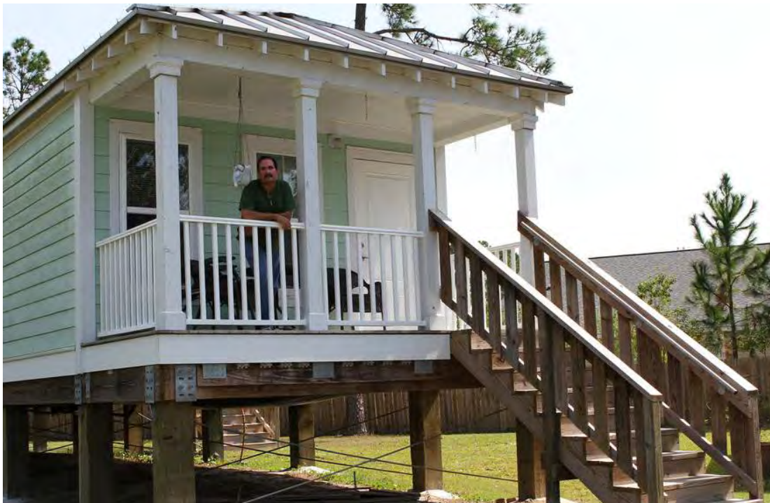
Figure 41: Katrina Cottage Weathers Hurricane Isaac, - Sep 20, 2012
