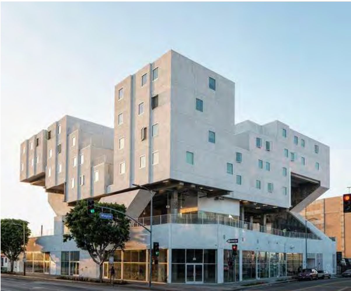
LA's Star Apartments: modular and prefabricated, six-storey residence built for Skid Row Housing Trust, LEED Platinum pending. Photo used with permission from Gabor Ekecs.
