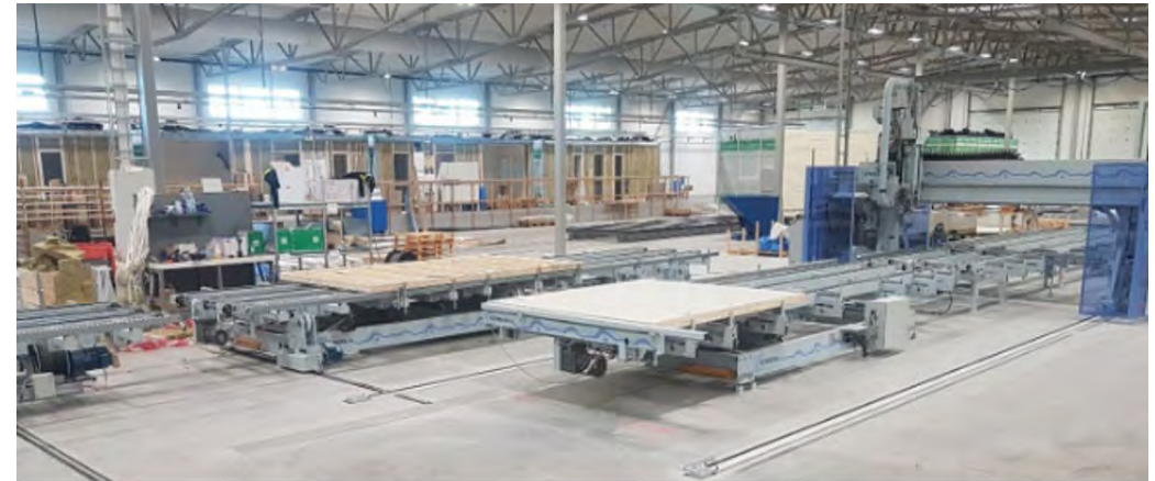
Prefabrication facility (Source: BC Housing)
