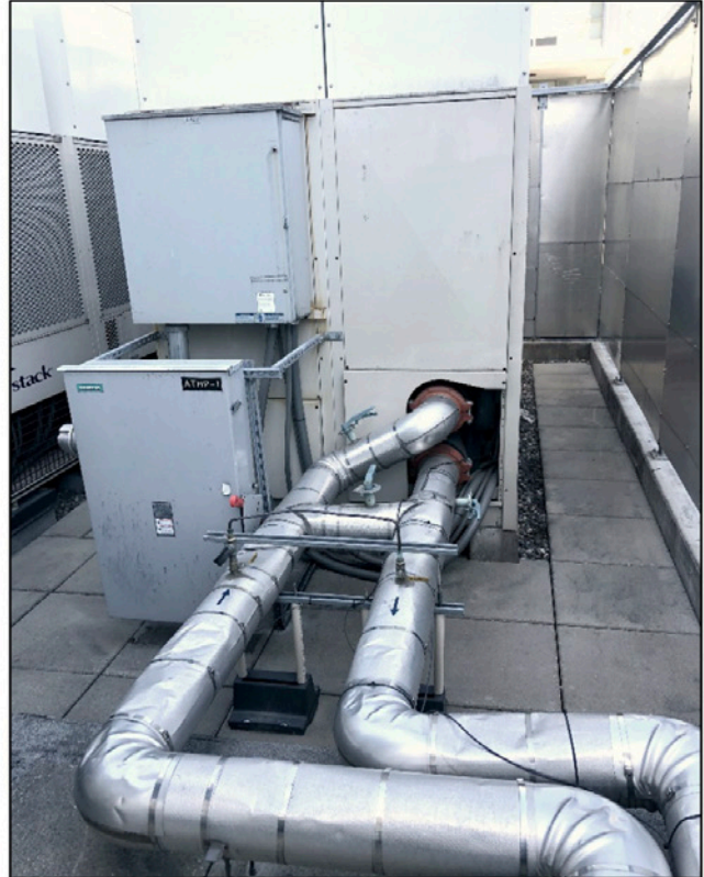
1249 Howe St. Air-to-water heat pump chiller. ATHP-1 - Airstack ASP 060X-H (2 modules)
