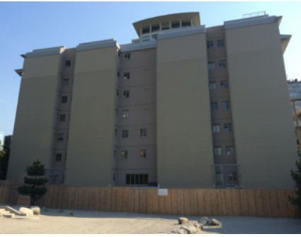
Brookland Court. 78 units - 7-storey senior development. Building envelope retrofit
