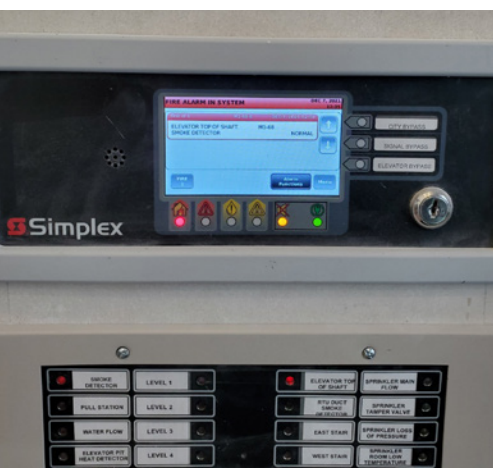
Inclusion Homes. 4872 Ontario Ave., 4897 Ontario Ave., Powell River. Integration system testing
