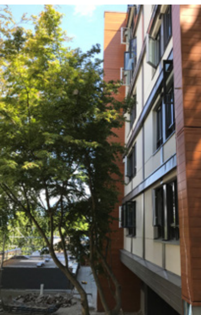
Grandview Terrace. Building envelope upgrade
