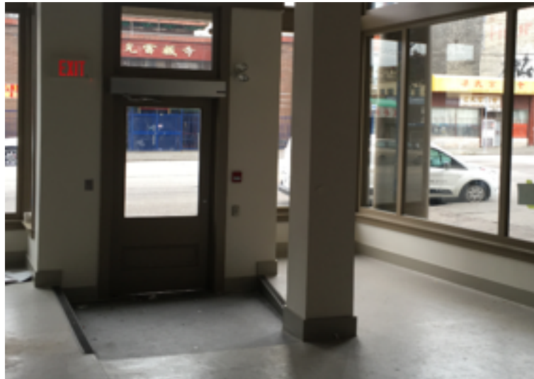
The Hazelwood, 342 East Hastings, Vancouver – recessed 1-2 inches inside CRU doorway for future “Pedestrian mats”
