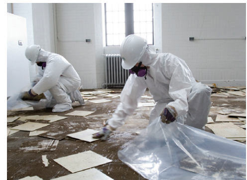
Workers removing vinyl-asbestos tiles.
